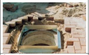
**Step 3** Insert lid. Screed sand, lay and cut pavers as normal.
