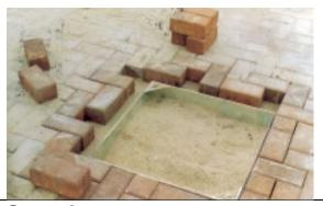
**Step 4** Fill Joints with dry sand. Compact carefully in the usual manner.
